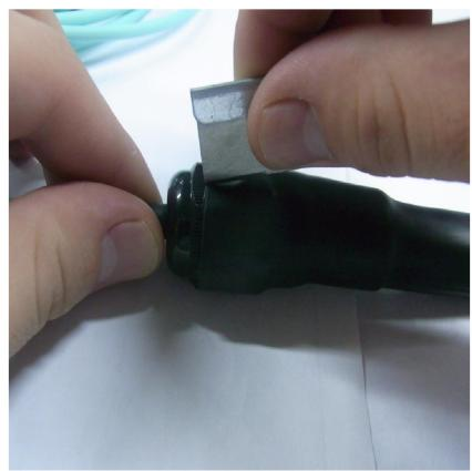
Use the knife to cut open the outer heat shrink tube.
